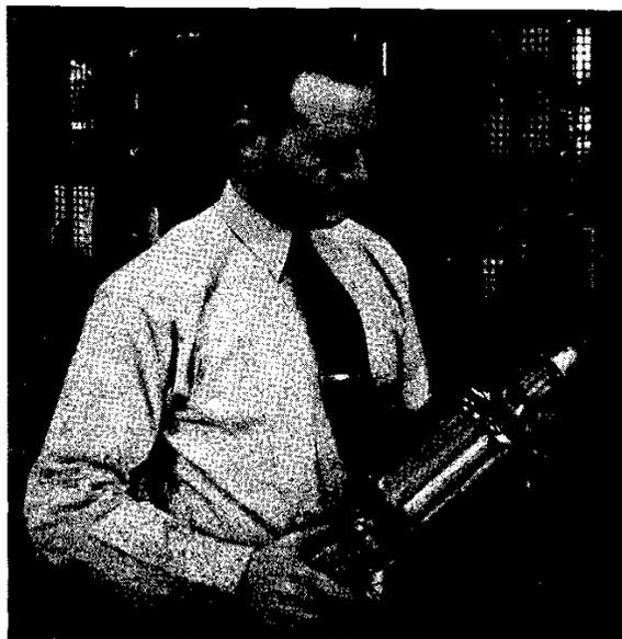
Walter W. McCoy, chief engineer of station WJAS, Pittsburgh, Pennsylvania, holds a 279A vacuum tube which was removed from the station's transmitter after 16,297 hours of operation. Although still functioning it was removed at the end of this period because the station feared it might fail and cause lost time on the air.
